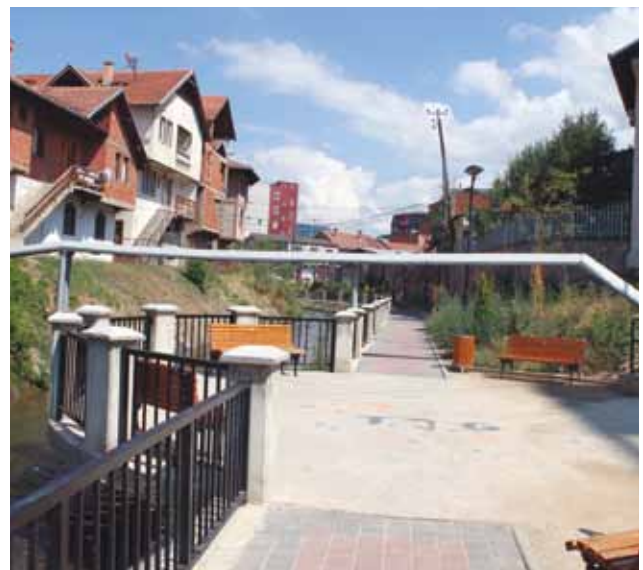
Project site 2: After
