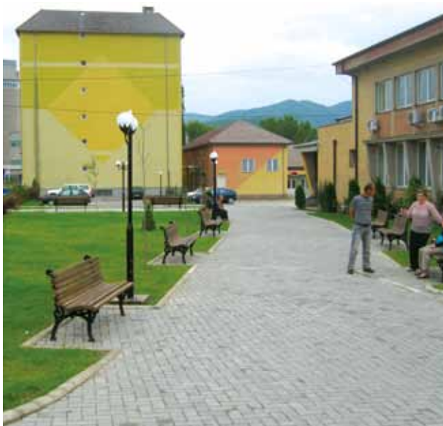
Project site 1: After
