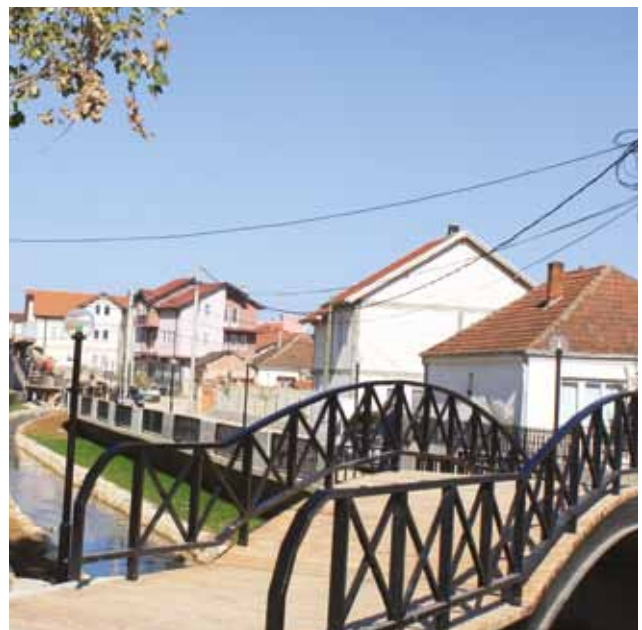
Project site 2: After
