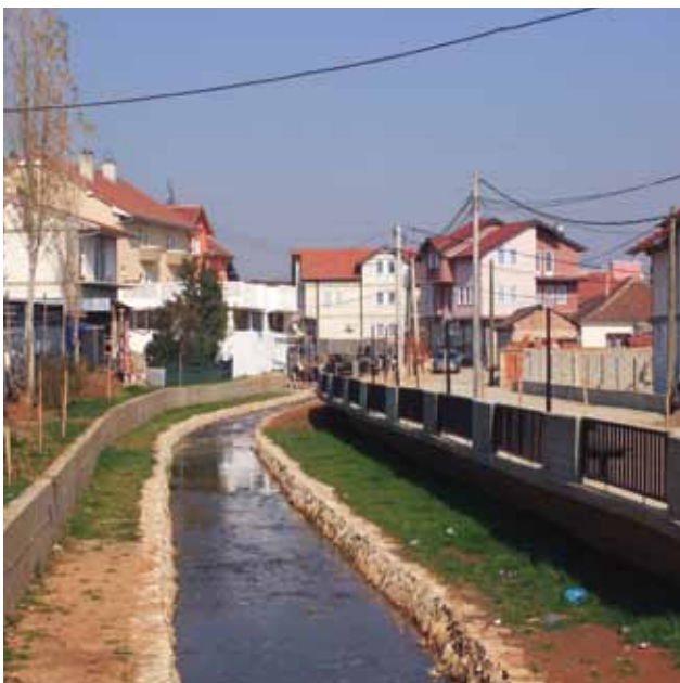
Project site 1: After
