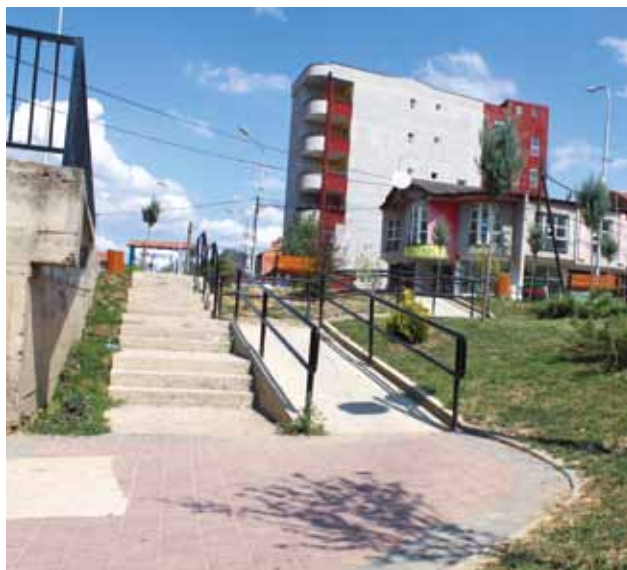
Project site 1: After
