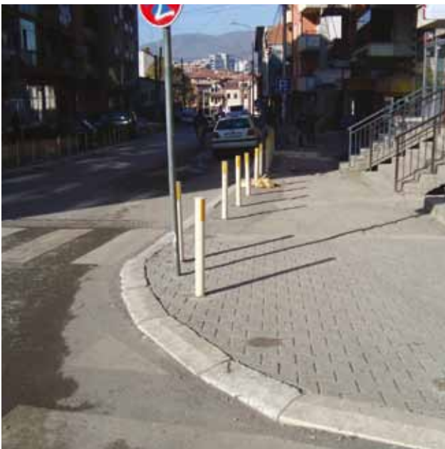
Project site 1: After
