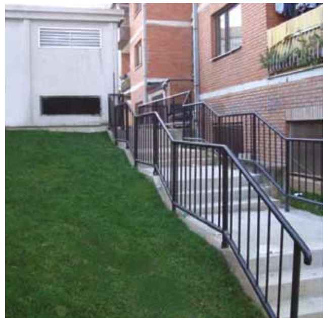
Project site 2: After
