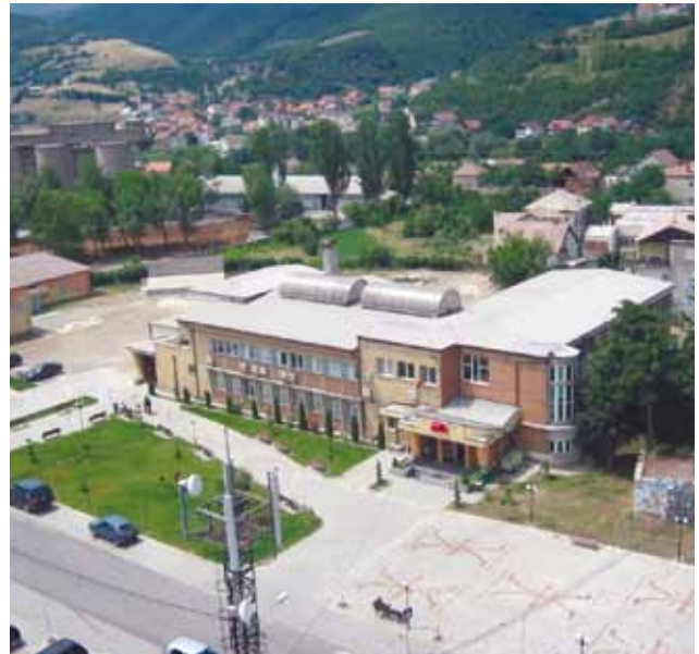
Project site 2: After
